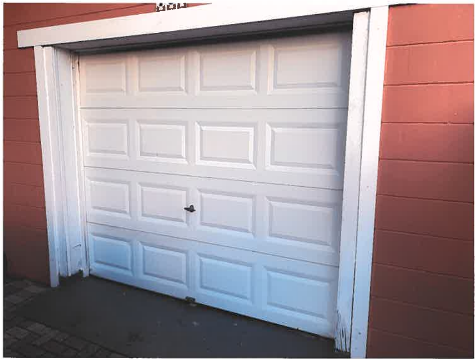
Photo 1A - Existing Garage Door West Elev (Toward Alley)
