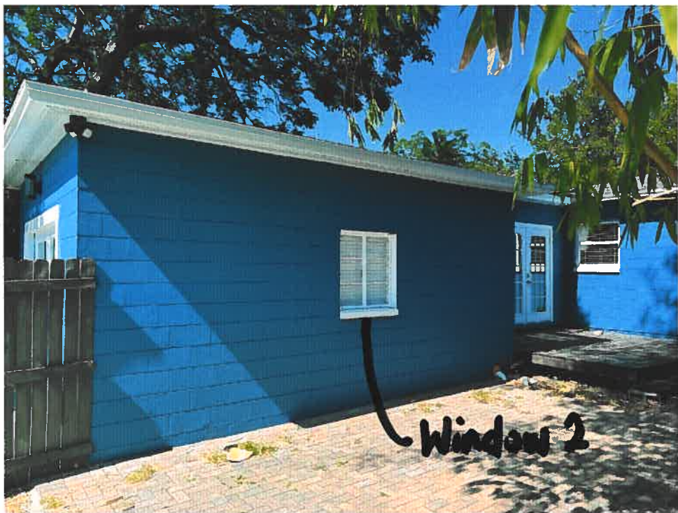
Photo 2 - So. Elevation Window 2
