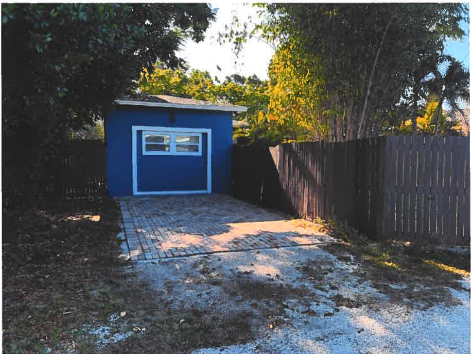
Photo 5A - Fence Photo A West & North Elevation
